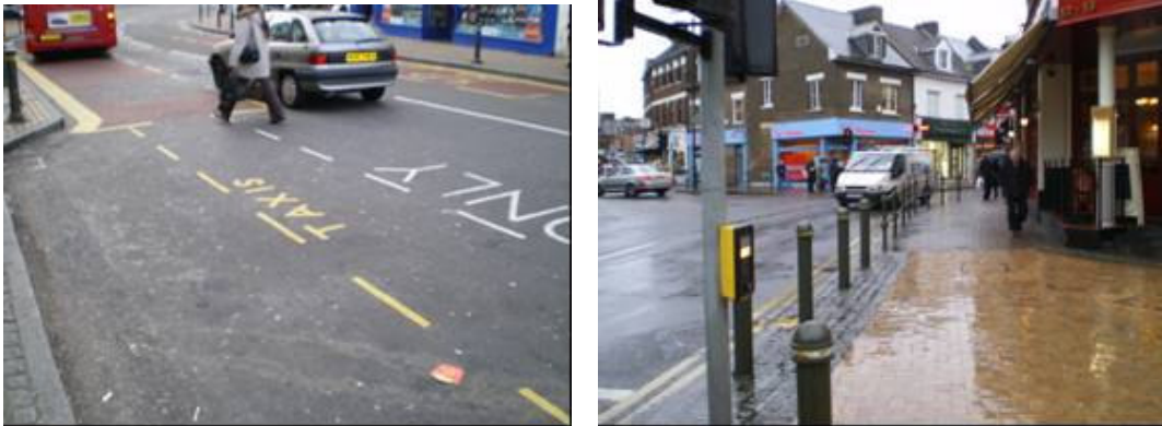
Figure 3.2: Road markings / bollards
