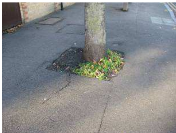
Figure E.17: Footway surface
