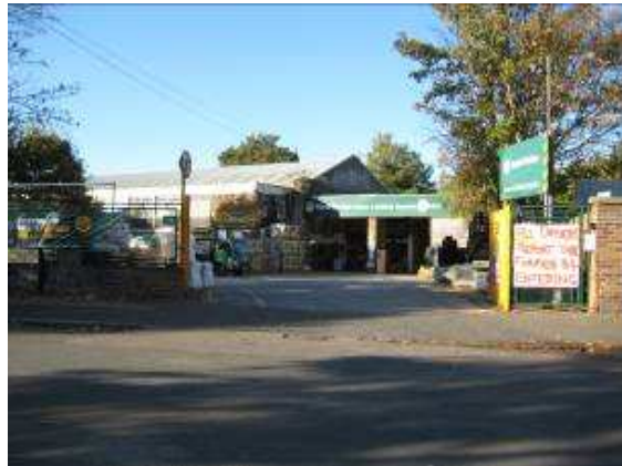
Figure E.12: Travis Perkins service yard entrance
